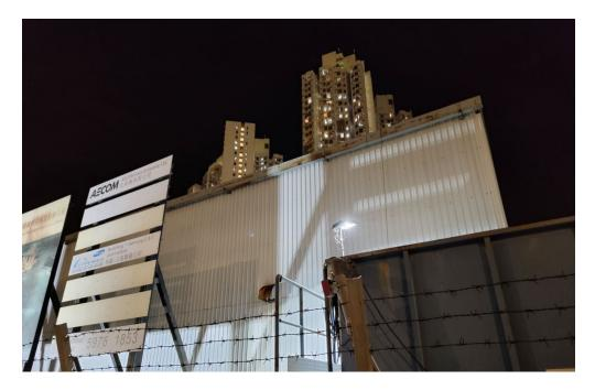
Photo 4 – Control of night-time lighting using light hooding
